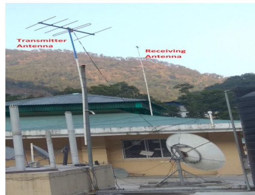
Fig. 6. Transmitting and Receiving antennas fitted onto the rooftop of the 5G_IoT Lab having the OTA range of 20 meter.
